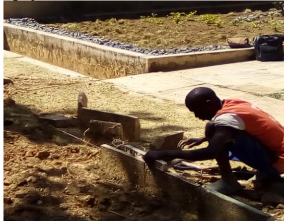
Plate xv: Laying of kerbs to define pedestrian walkway
