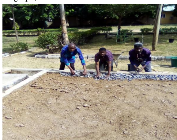
Plate iii: Laying of gravels and stone pebbles For demarcation and emphasis
