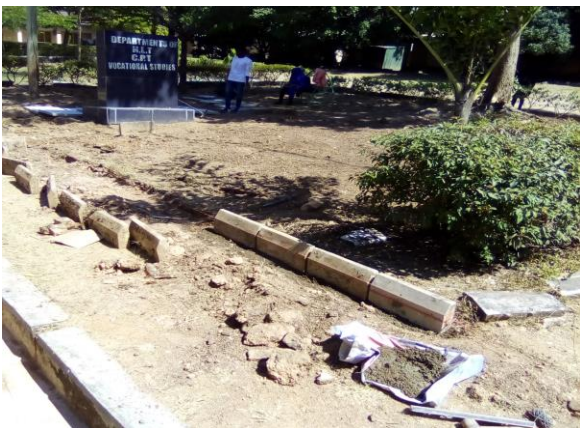
Plate viii: Site clearing, weeding and disposal
