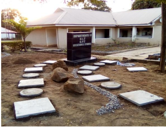
Plate x: Laying of concrete floor slabs, stone Chippings (Gravel) and rock boulders As pedestrian walkway to sit-outs
