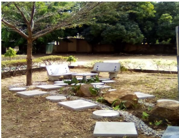
Plate xiv: Installation of concrete table and chairs
