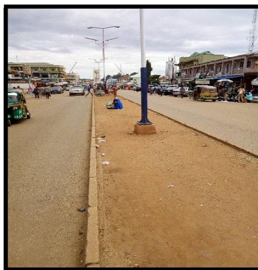
Figure 6: Absence of Softscape Elements on Road Verge .Source: Researchers' Field Survey, 2019
