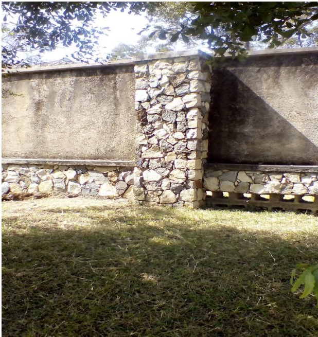
Plate xv: A mortared stone wall made from Limestone used for fencing at G.R.A. Jos.
