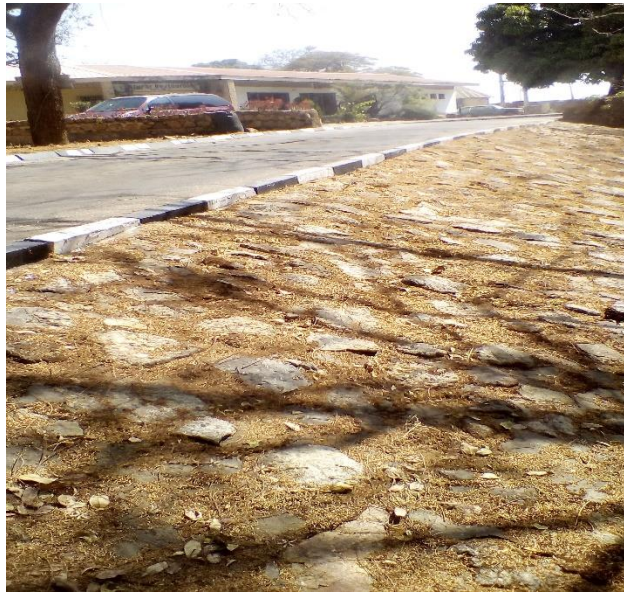
Plate xvi: Use of stones for sloppy terrain Source: Author's field work, 2019.
