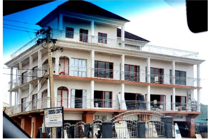
Fig. 16 Commercial complex in Kaduna South, Sabo
