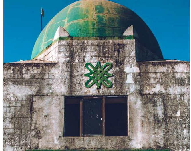
Fig. 6 Lugard Hall building showing dome and pinnacle
