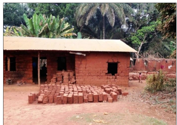
Fig 12:- Rectilinear building construction in Igala Land, with mud bricks, corrugated iron roofing sheets. (Source: - Emusa, 2018.)
